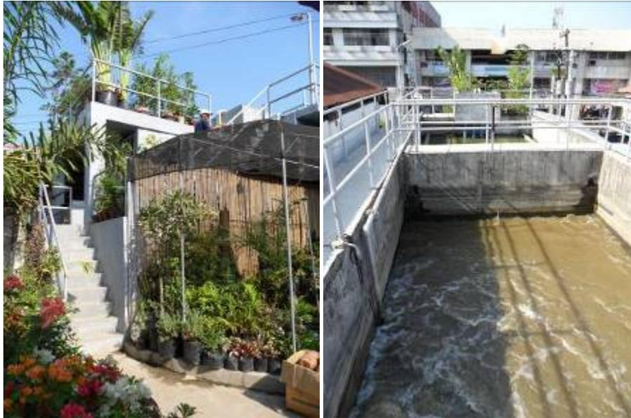
**Figure 2.** The San Fernando Market wastewater treatment plant (left) and its SBR and UASB (foreground/background, right)
